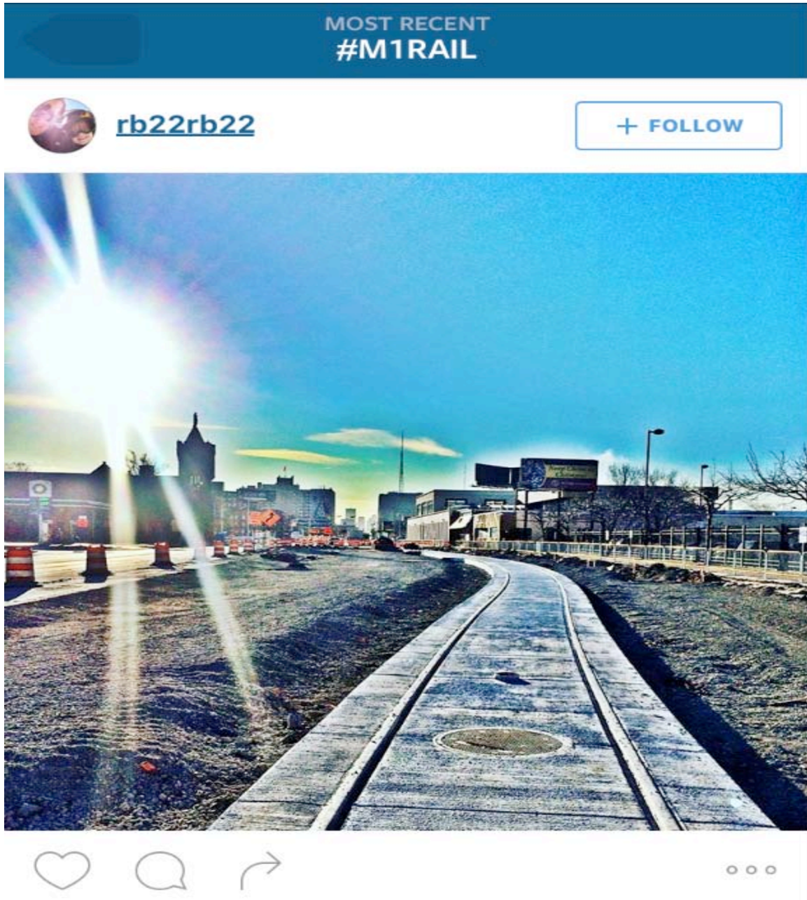
This is a photo from the M1 Website showing the new rail tracks curving right in front of Rosary!
