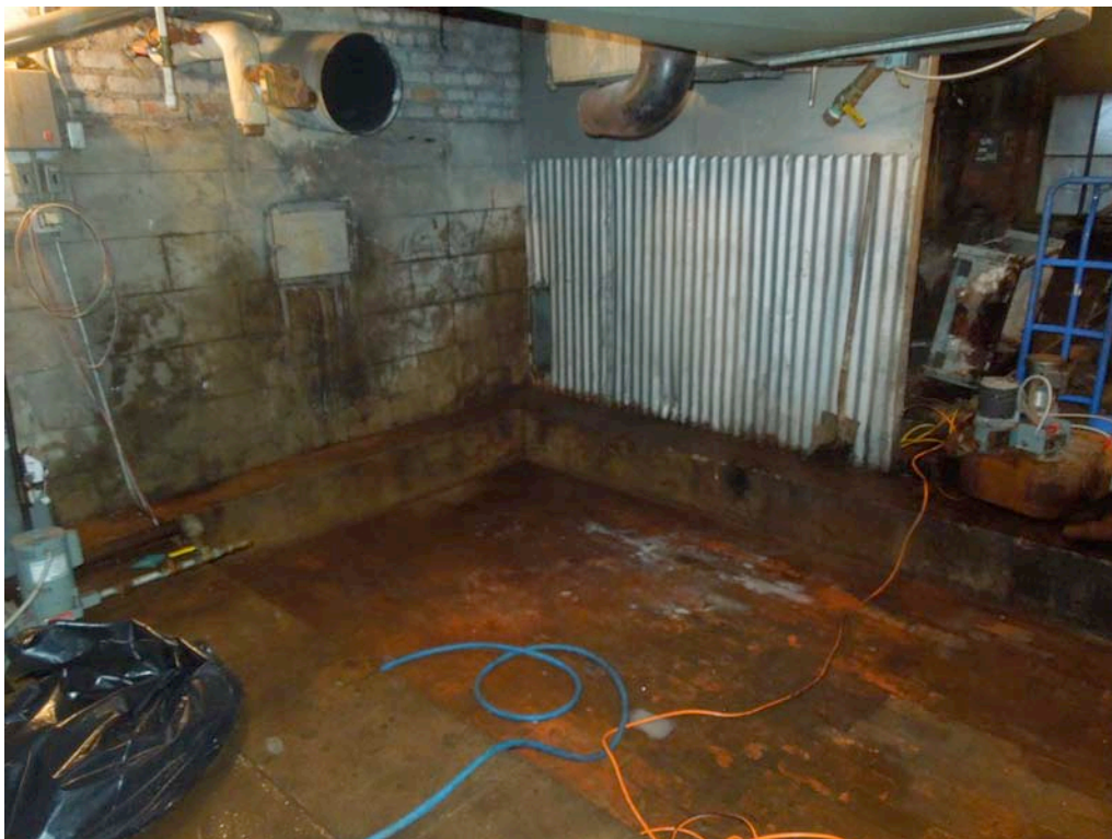
The same view with the boiler removed.
