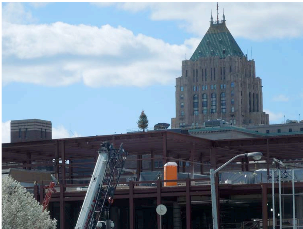
It would be easy to miss the one lonely evergreen tree on the top of the new Wayne State building across the street. This is the traditional “topping” of construction indicating the builders have raised the structure to the highest level planned.
